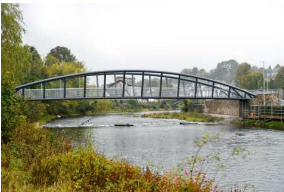
Figure 3: Gooseholme Bridge, Kendal
