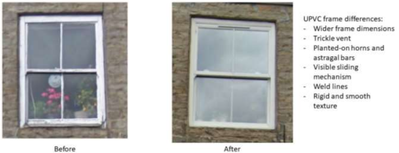
Figure 139 Differences between timber and uPVC sash windows
