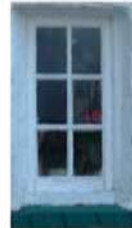
Many 16 and 17 century formerly leaded or unglazed windows have now been replaced with timber windows
