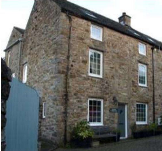
Figure 12 Blocked first floor opening and external stairs removed
