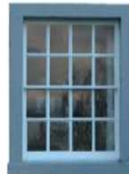
Late 18 early 19 century 16-paned Georgian sash - without horns
