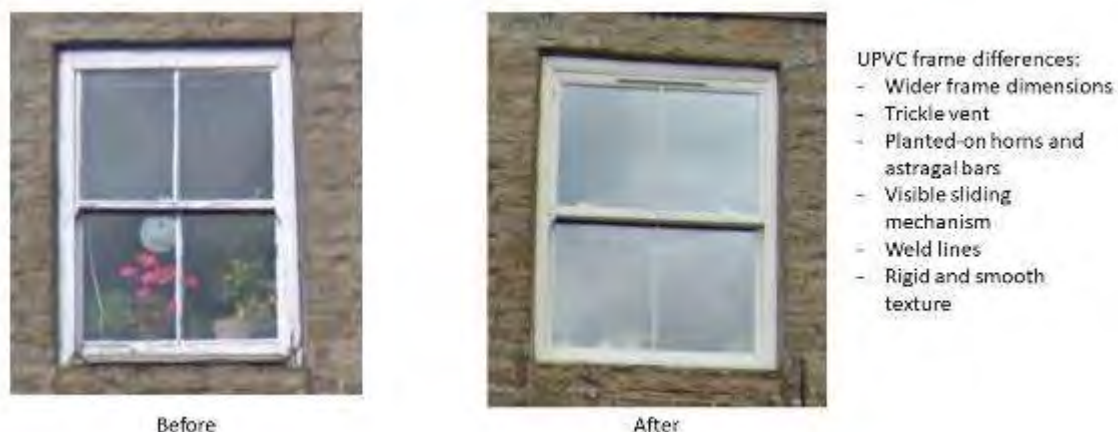
Figure 138 Differences between timber and uPVC sash windows
