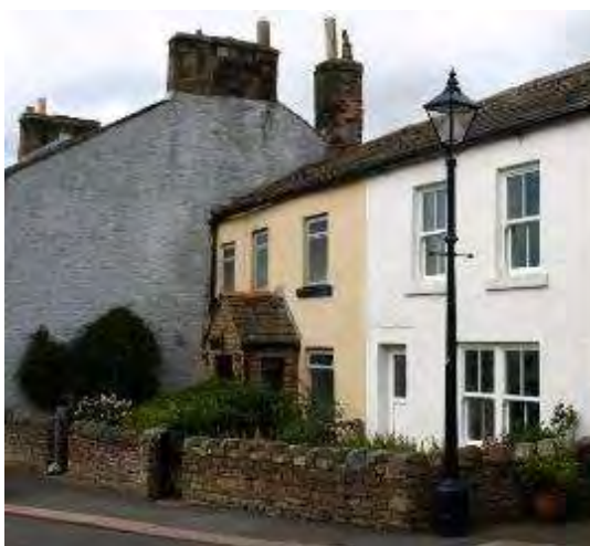
Figure 33 Rubble garden wall with saddleback coping stones
