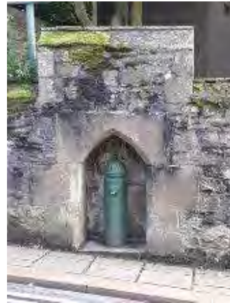
Figure 44 Standpipe
