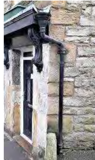
Figure 20 Cast-iron hopper and downpipe
