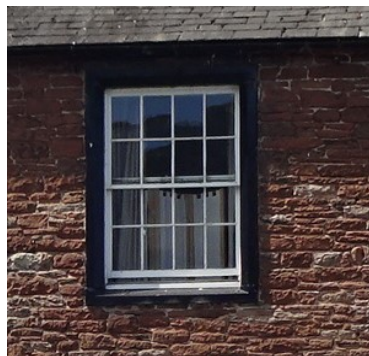
Figure 10 8x8 sash window
