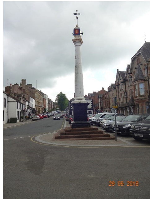
Figure 69 Low Cross (prior to repair)
