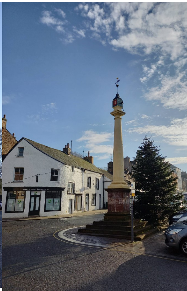
Figure 124 Low Cross following repair works
