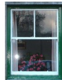
Late 19/early 20 century sash
