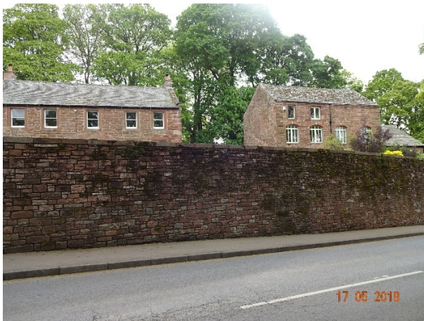
Figure 114 The former brewery buildings (also referred to as Bobbin Mill)
