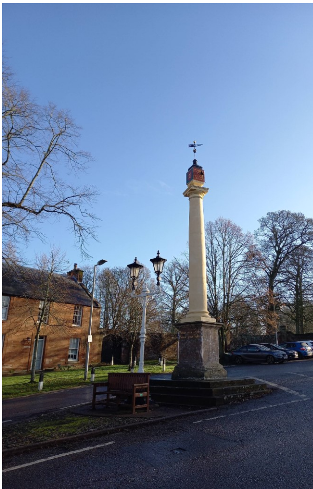
Figure 123 High Cross following repair works
