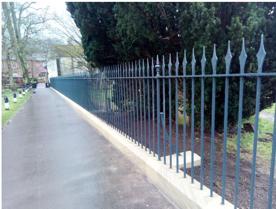
Figure 125 New railings around St Lawrence's churchyard
