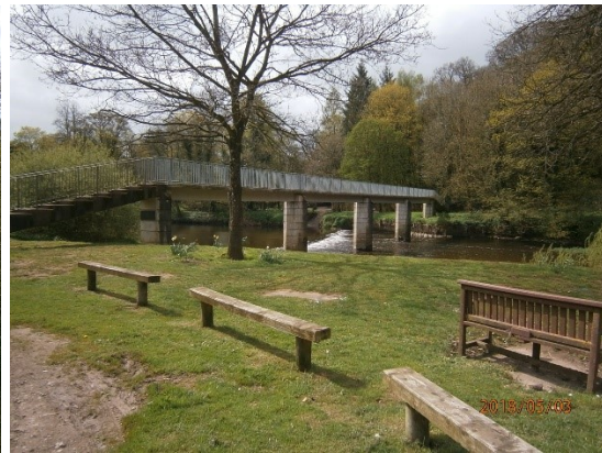
Figure 94 Jubilee footbridge replaced in 1970
