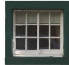
Early 18 century horizontal sliding sash or 'Yorkshire Lights', often found in cottages
