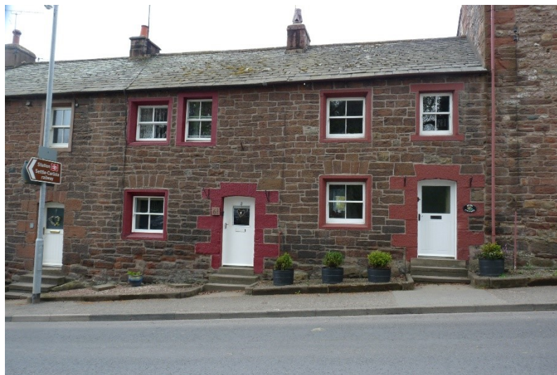
Figure 78 Buildings with deep set chamfered windows
