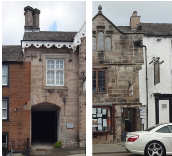
Figure 64 The over-key of quoins is evidence of attempts to unify building lines
