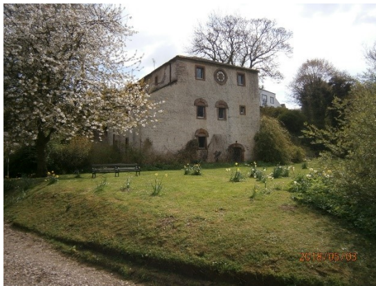
Figure 93 Bongate Mill (grade II listed)
