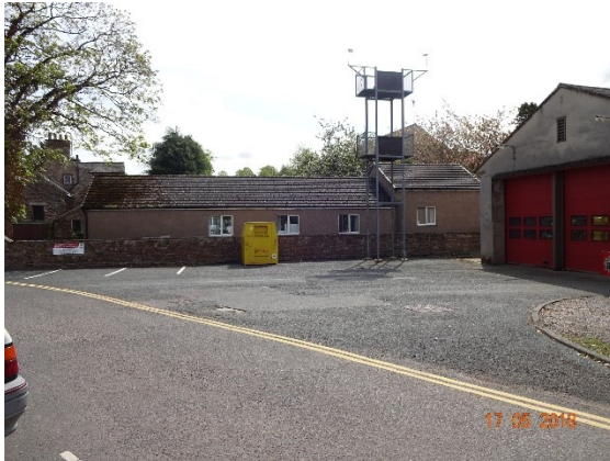
Figure 52 Fire station and Guides hut
