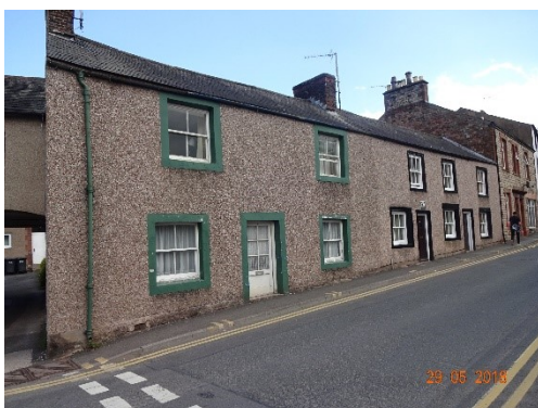
Figure 54 Smaller residential properties to western end of High Wiend
