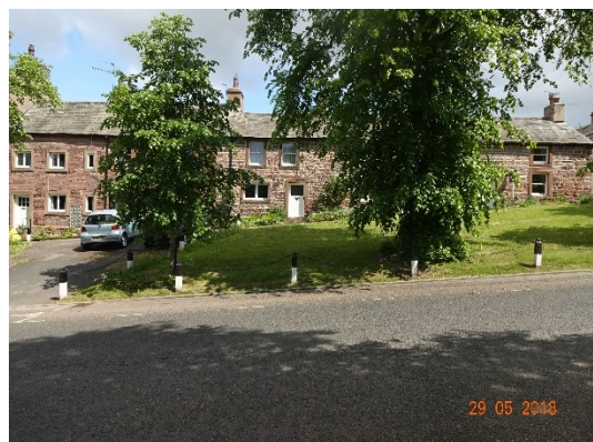
Figure 67 Vernacular buildings on the eastern side of the street
