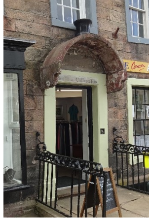
Figure 8 Hoodmould
