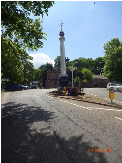
Figure 68 High Cross (prior to repair)
