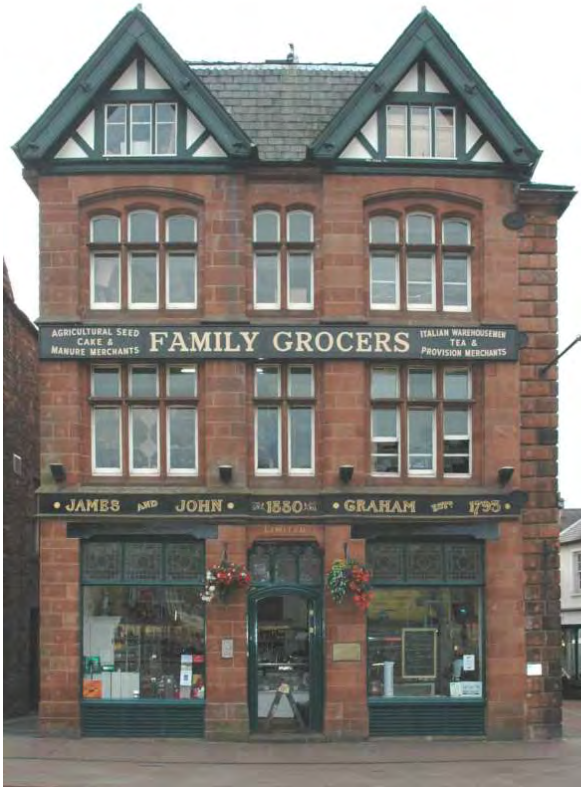
J & J Graham. Building with integral shopfront c1880
