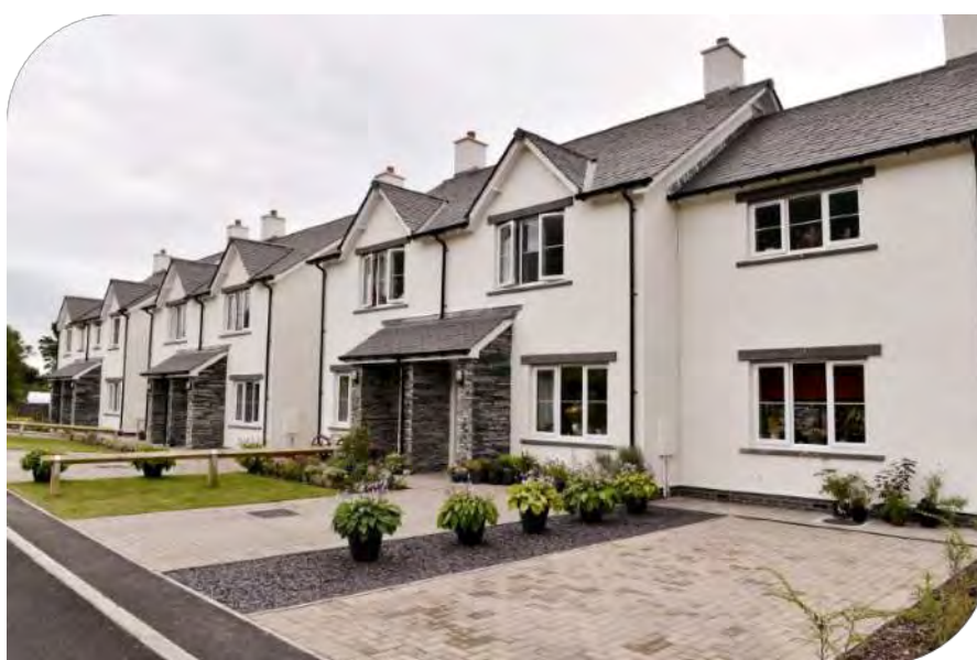
Spring Close, Threlkeld – recent development of affordable housing by Eden Housing Association
