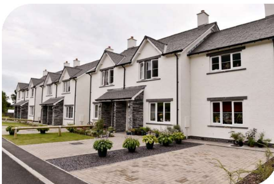
Spring Close, Threlkeld – recent development of affordable housing by Eden Housing Association
