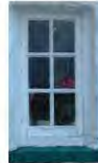
Many 16 and 17 century formerly leaded or unglazed windows have now been replaced with timber windows
