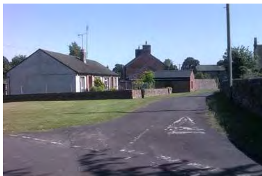
Figure 25 Informal road verges at junction to Church Lane
