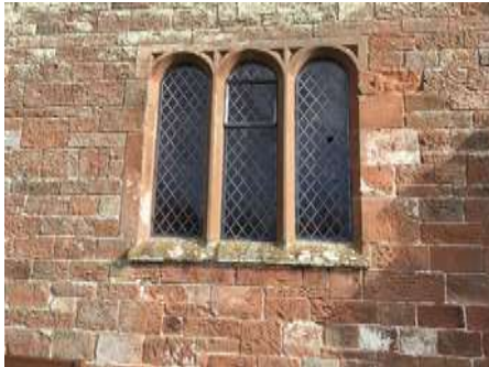
Figure 11 Cracked glass in south elevation window of St Oswald Church
