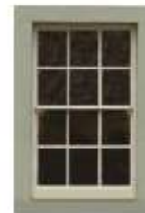
Early 18th century 12-paned Georgian sash - without horns
