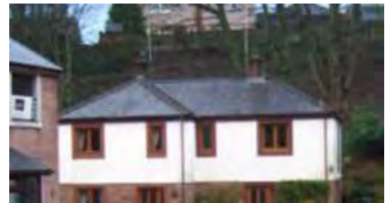
Figure 3 Modern house with slate roof
