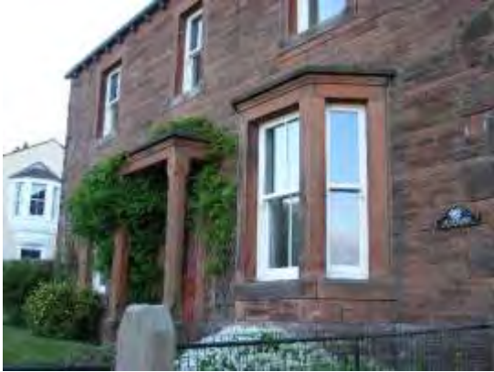
Figure 12 This house has a number of decorative flourishes. Note the projecting bay window, the pillared porch, the emphasised quoins at the corners of the house, and the dentillation at the eaves. There is also an angular sandstone gatepost in the foreground
