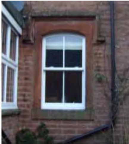
Figure 20 Ornate window with moulded hood
