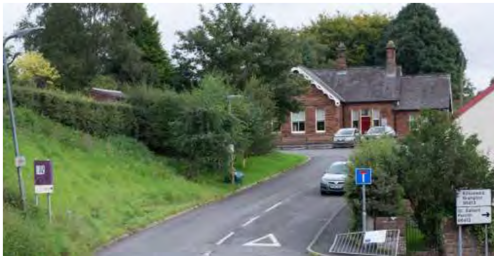
Figure 4 View towards the railway station
