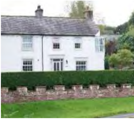
Figure 9 Unusual, almost bartizan-type window turret
