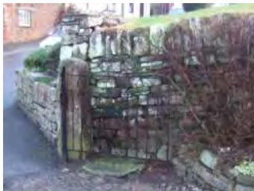
Figure 26 Sandstone wall with rounded capping, simple sandstone gate-post with rounded top
