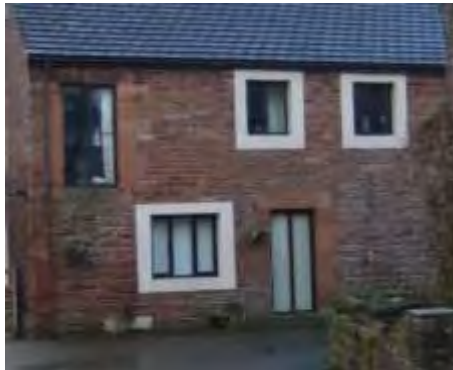
Figure 21 Modern barn conversion, windows have simple sandstone surrounds with the majority painted
