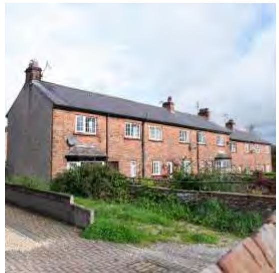
Figure 37 Terrace of recent houses opposite the Village Hall with sandstone facades and rendered gables
