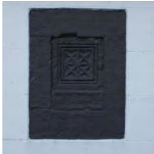
Figure 15 Decorative inset from the wall of the fire-station
