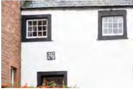
Figure 36 Rendered façade of house of 1617 with small windows and date-stamp above door
