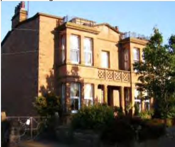
Figure 13 House in the style of a Victorian villa with projecting bays, a connecting balcony at first-floor level and a pedimented central bay
