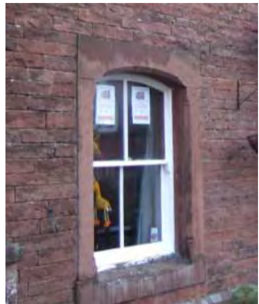
Figure 19 Typical window with sandstone surround and two-over-two sliding sashes
