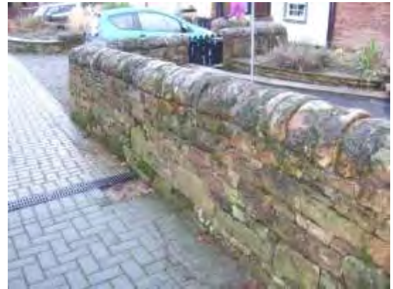
Figure 27 Sandstone wall with rounded capping
