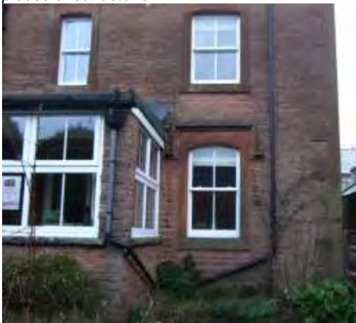
Figure 18 Another typical village house of rough-dressed sandstone ashlar and dressed ashlar to emphasise the corners of the main house. The front extension is not of the same quality
