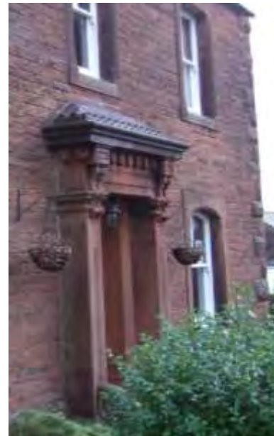
Figure 11 Decorative door surround with Classical styling, the corner of the house has emphasised quoins, in the background
