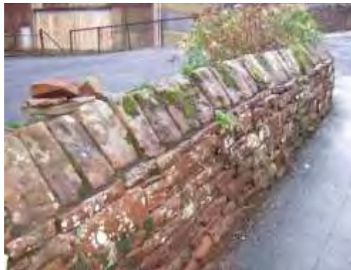
Figure 24 Sandstone wall with triangular capping
