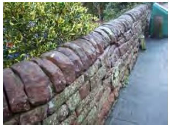
Figure 28 Sandstone wall with rounded capping
