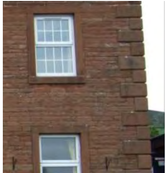
Figure 10 V-jointed sandstone quoins
