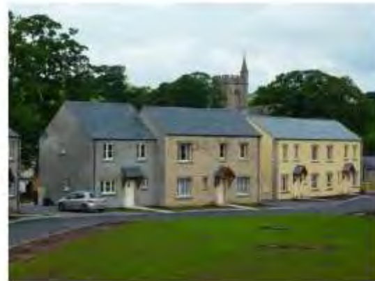
Photos courtesy of Westmorland Gazette and David Graham
