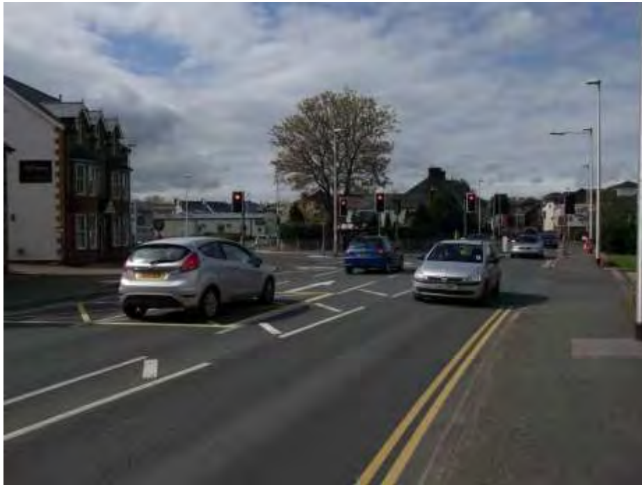
Figure 5 Junction with Victoria Road and Southend Road
