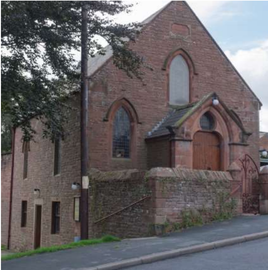
Fig 17 Former Methodist Chapel, potential location for café
