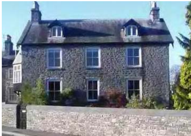
Victorian building - Coldbeck House
