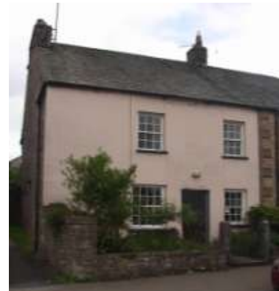
Simple plain front facades Timber vertical sliding sash windows
