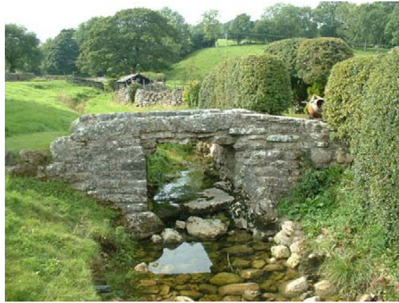
Limestone footbridge over Dale Beck by Ash Croft
