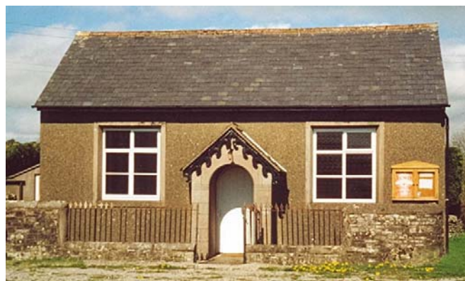
Carved bargeboard, low limestone wall and railings - Methodist Chapel
