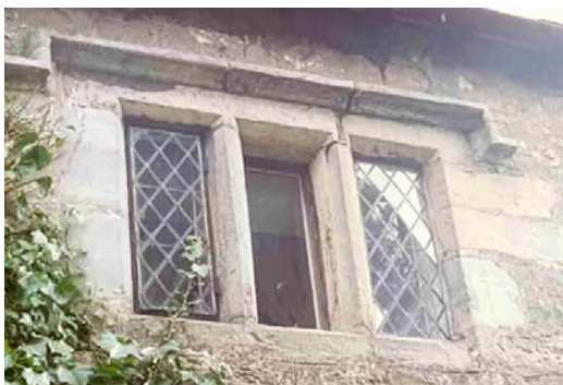
Casement windows and stone mullions (Old Rectory)
