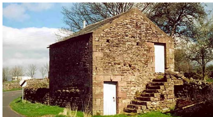
External stone stairs
