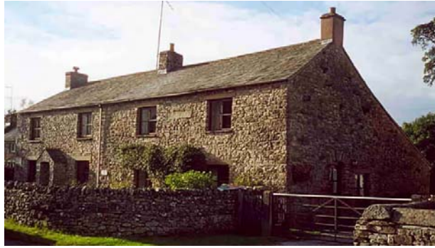
Stained casement windows and rear outshut roof at Harlea House
